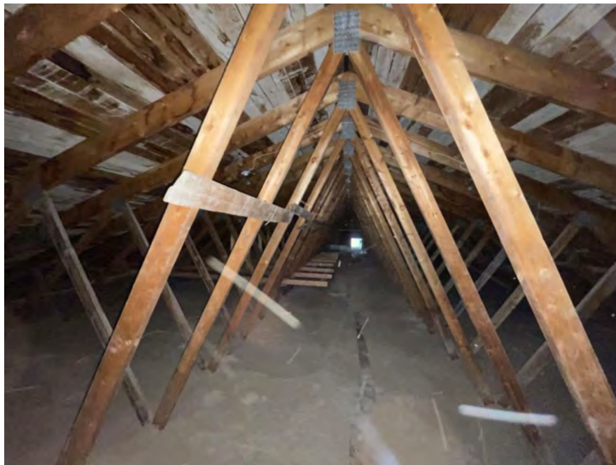
Figure 2: Typical roof truss.
